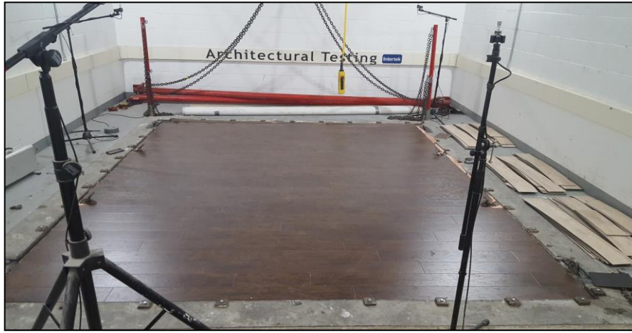
Source Room View of Test Specimen Installation
